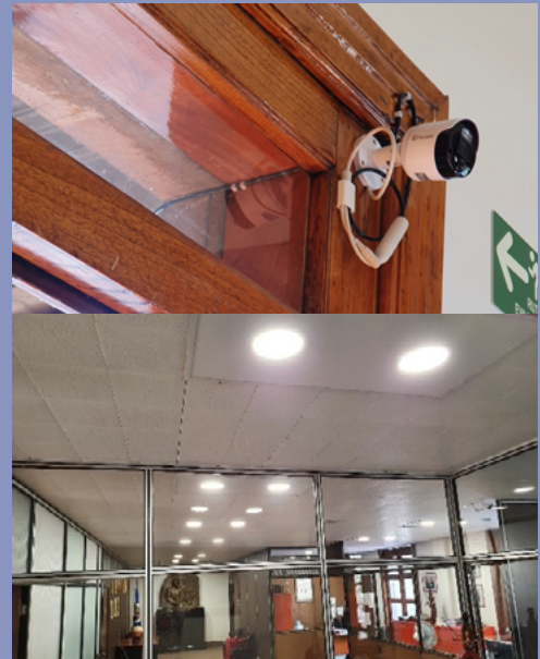
Installation of the video surveillance system and LED luminaires
